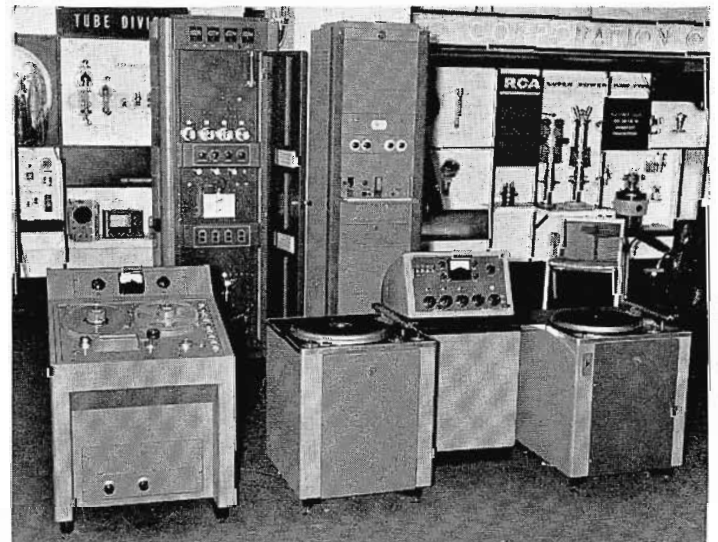
RCA AUDIO EQUIPMENT FOR AM/FM AND TV STATIONS . . . In the foreground (l. to r.) is an RCA console mounted tape recorder and two new BQ-2A Turntables flanking a BC-4A Audio Central. Cabinet racks house (left) a 250 watt AM Transmitter, and (right) a new line of printed circuit audio amplifiers.
