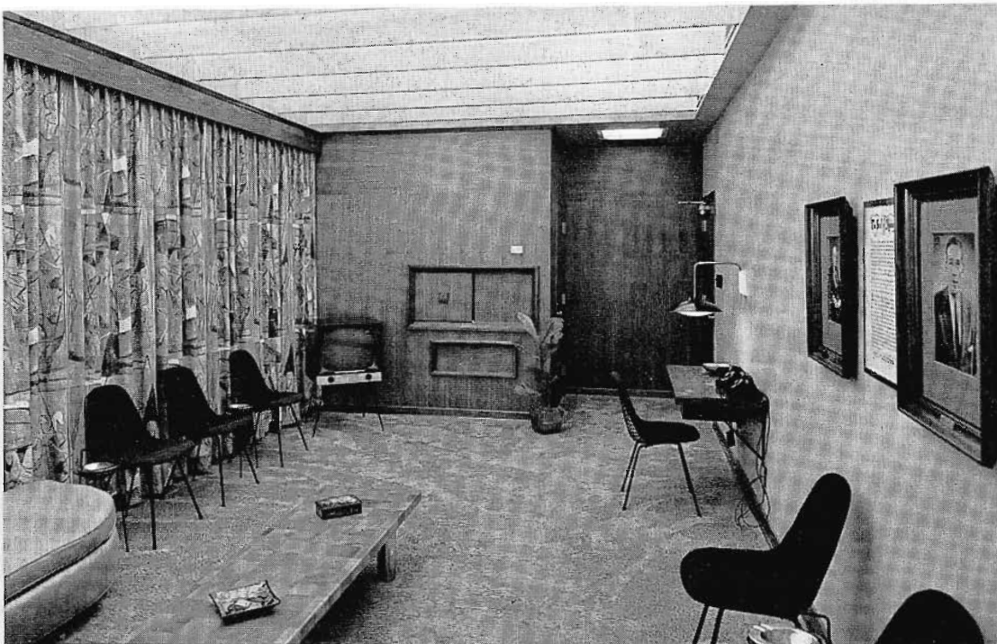
FIG. 16. This spacious and well-appointed conference room adjoins the manager's office in the new WHIO Building. The lighting system is unusual. Two 6-foot slimline tubes have been installed end-to-end and are supported by special steel channels which extend from wall to wall at 2-foot intervals. The channels also support V-shaped, perforated metal acoustic baffles. By mounting the tubes 18 inches below the reflective ceiling and operating them through remote ballasts, which are easily accessible on the opposite face of the wall shown here on the right, the engineers provided ideal lighting and eliminated any possibility of operating noise.
