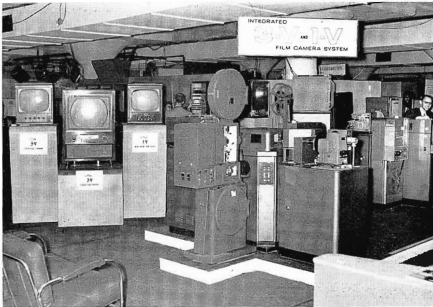
INTEGRATED 3-V AND 1-V FILM SYSTEM . . . The new RCA TP-15 Universal Multiplexer was the hub of this film system for both color and monochrome. A 21 inch color receiver (center) displayed pictures from the 3-V camera, the utility monitor (left) showed the compatible monochrome picture from the 3-V, and utility monitor (right) showed the output of the 1-V monochrome film system.
