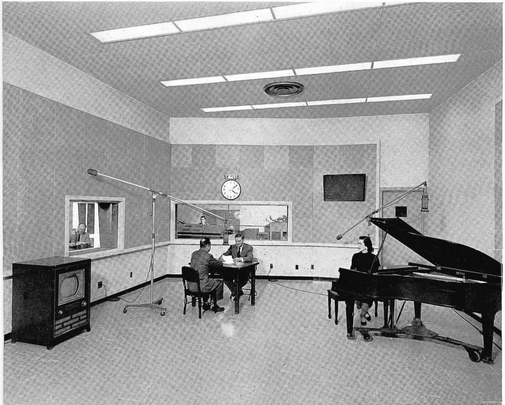
FIG. 13. WHIO's main AM studio. Walls are covered by perforated asbestos board which covers acoustical materials of various densities chosen to provide an ideal frequency curve. Smaller AM studio can be seen through window at left and AM control room through window at rear.
