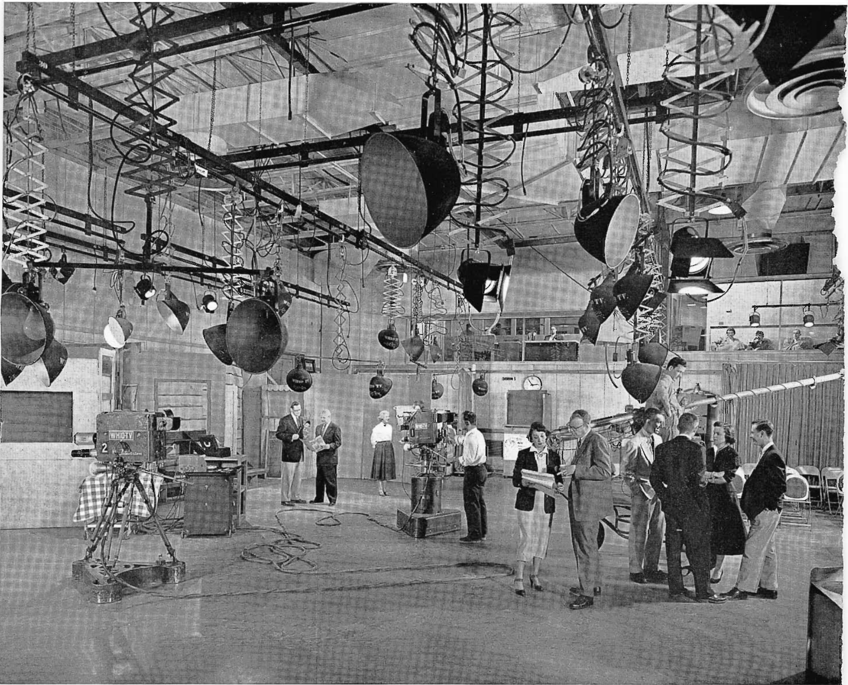
FIG. 5. WHIO's new TV studio is 50 feet wide by 63 deep. Elevated director's booth makes it possible to place sets around all four sides.
